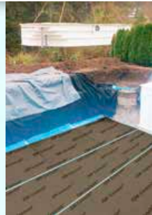
Conductive foil installation
