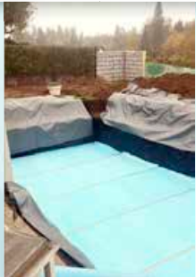
Preparing for installation
